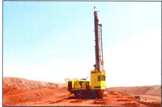
Photo 9 : Showing Drilling with dust extraction
