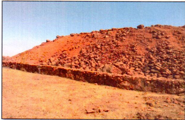
Photo 3: Showing Retaining Wall
