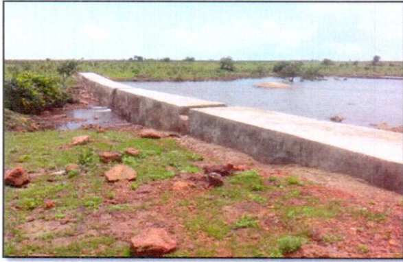
Photo 1: Showing check dam for water management
